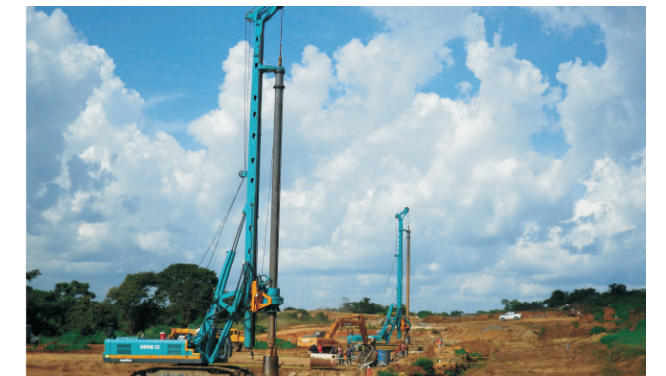
Construction of Tinaco-Anaco Railway - Venezuela
