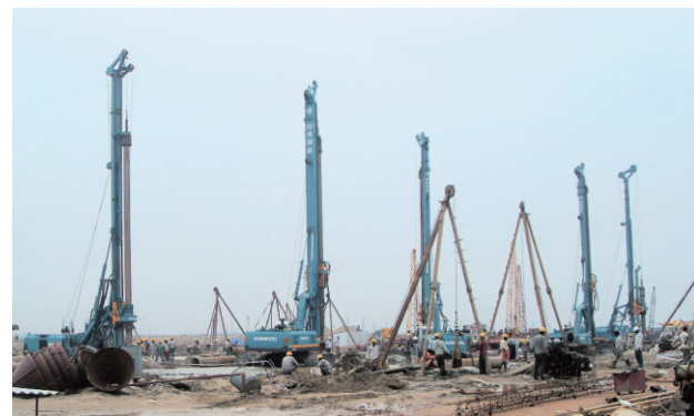
Construction job site - The Ganga River, India
