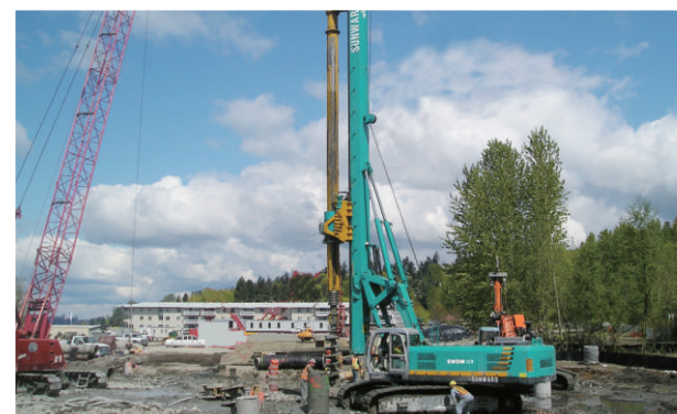
Construction job site - USA
