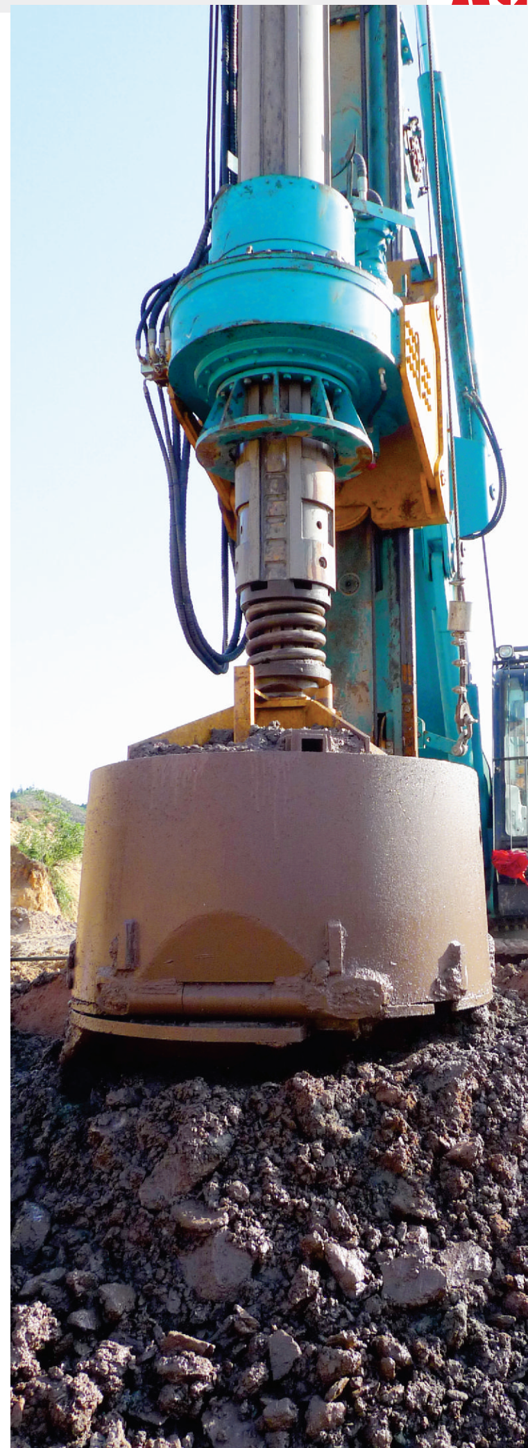
This is Feiyun river bridge construction in Wenzhou. In this project, the construction aperture is 2.2 meters and the depth is about 98 meters which is about 90 meters below the surface. Under the bottom of the sea surface is within 0 ~ 60 meters for silt layer, muddy clay layer, as well as 60 meters for gravel layer. Single-hole drilling a hole is about 7 hours.
