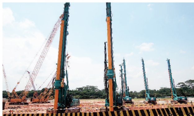
Construction of Metro - Singapore
