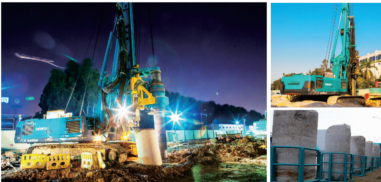
The maximum length of the rock core taken out of 1.95 meters and 1.2 meters in diameter in the Xiamen subway construction.
