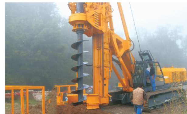
CFA Drilling - Switzerland
