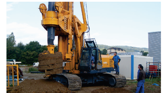
CFA Drilling - France
