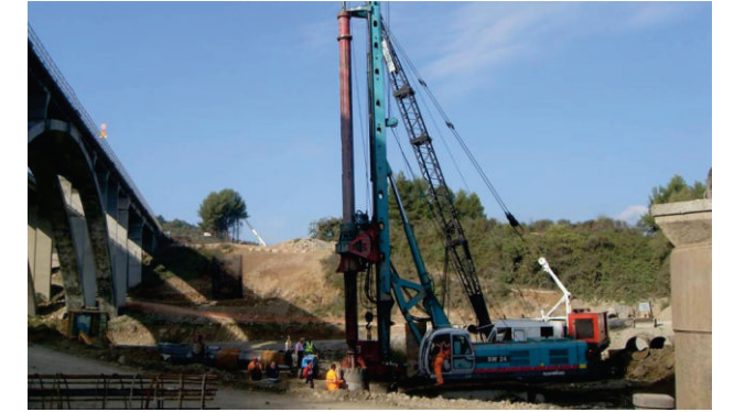
Salerno construction site, Italy
