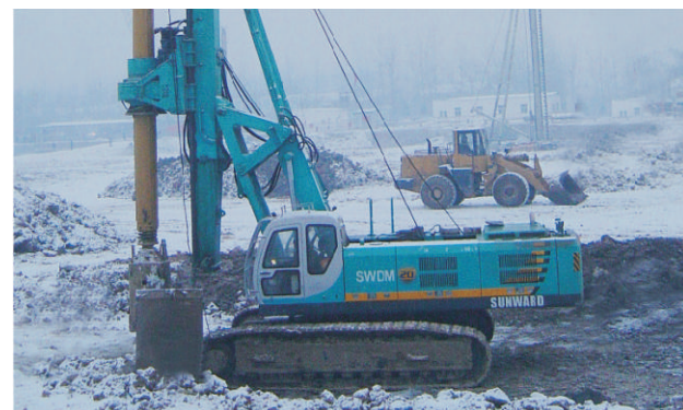
Construction site at -30 - Moscow, Russia
