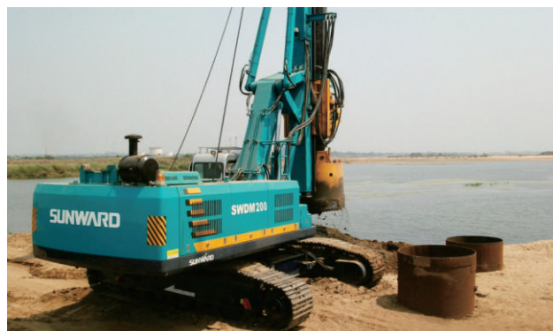
Godavari Bridge - India
